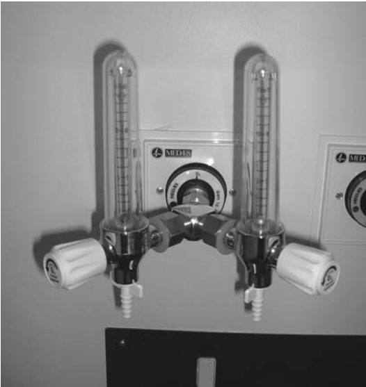
Figure 1.1 A wall mounted oxygen cylinder, fitted with a variable oxygen-flow-rate meter capable of delivering up to 15 litres/min
